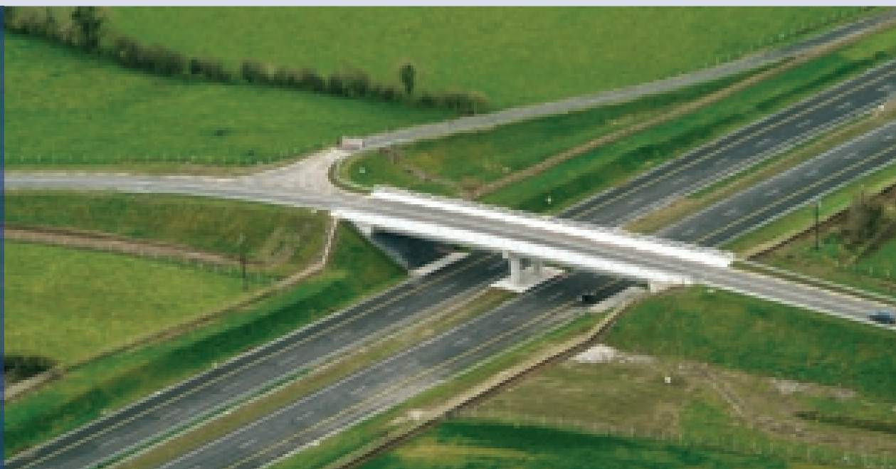
M4 Motorway, Completed, 2005
