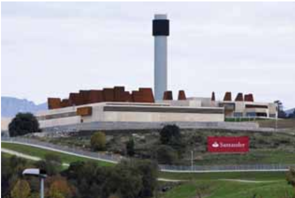
Data centre Cantabria
