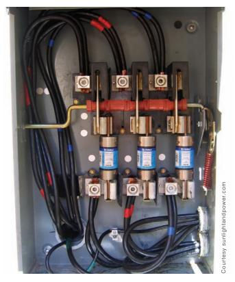
**PV** service disconnect A fused 3-phase safety switch serves as the PV service disconnect at a site employing a supply side connection. Note the use of paralleled conductors and lugs rated for two conductors each.
