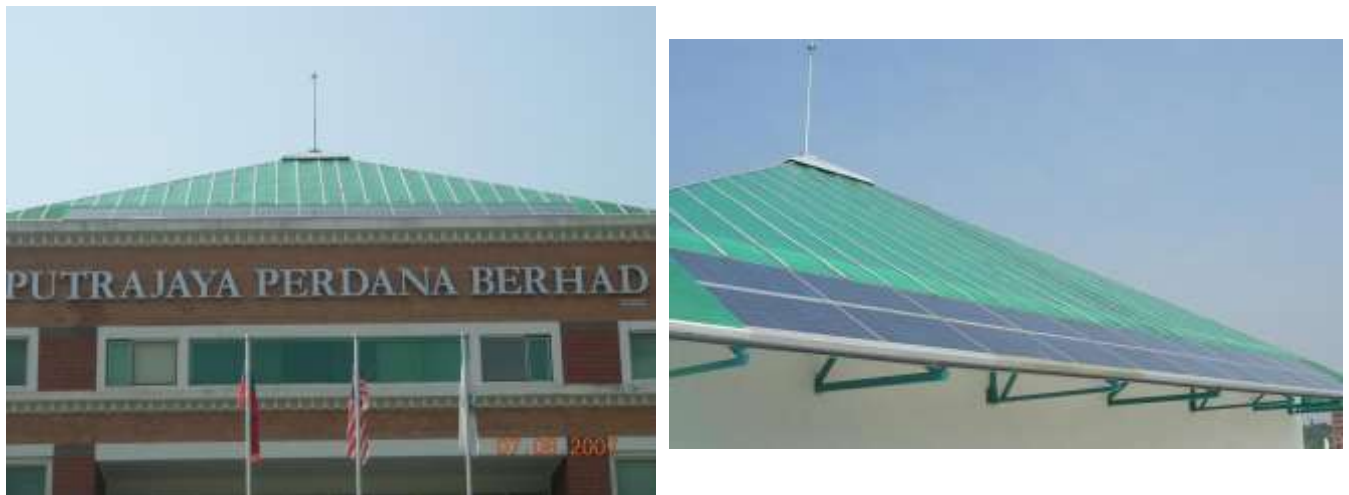
Figure 1: PV modules.
