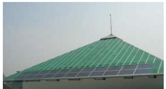
PV modules are nicely integrated into the existing polycarbonate roof.
