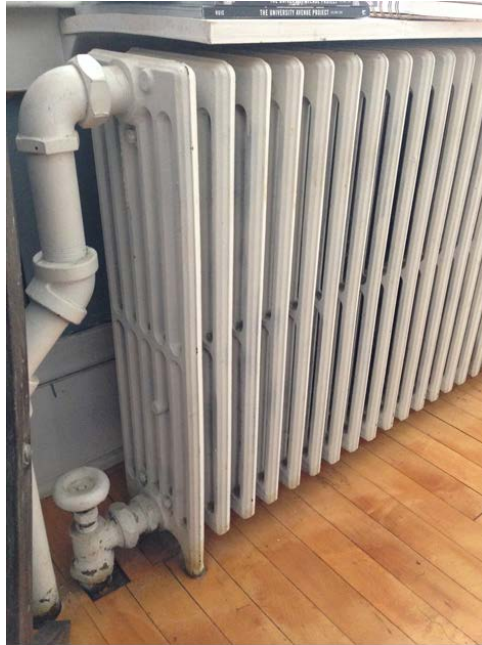
Figure 23. Tube style radiator, also called slenderized radiators
