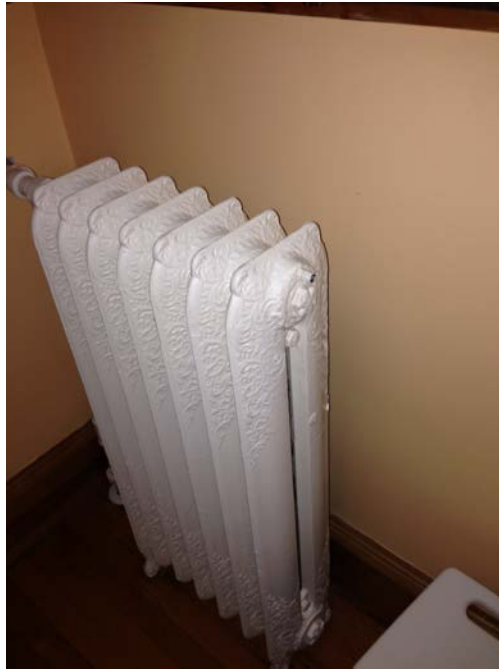
Figure 22. Three column cast iron radiator
