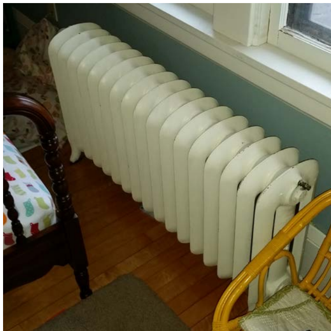
Figure 22. Three column cast iron radiator
