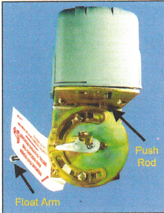
Starting Orientation of Float Arm and Push Rod
