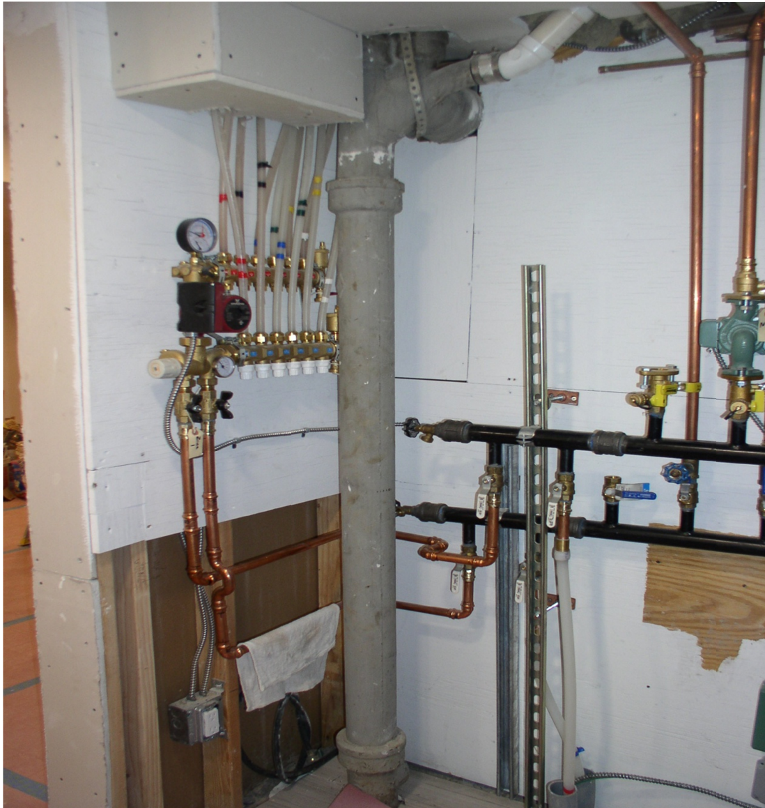
Zone 4 Main floor joist trac Caleffi 1725F1A
