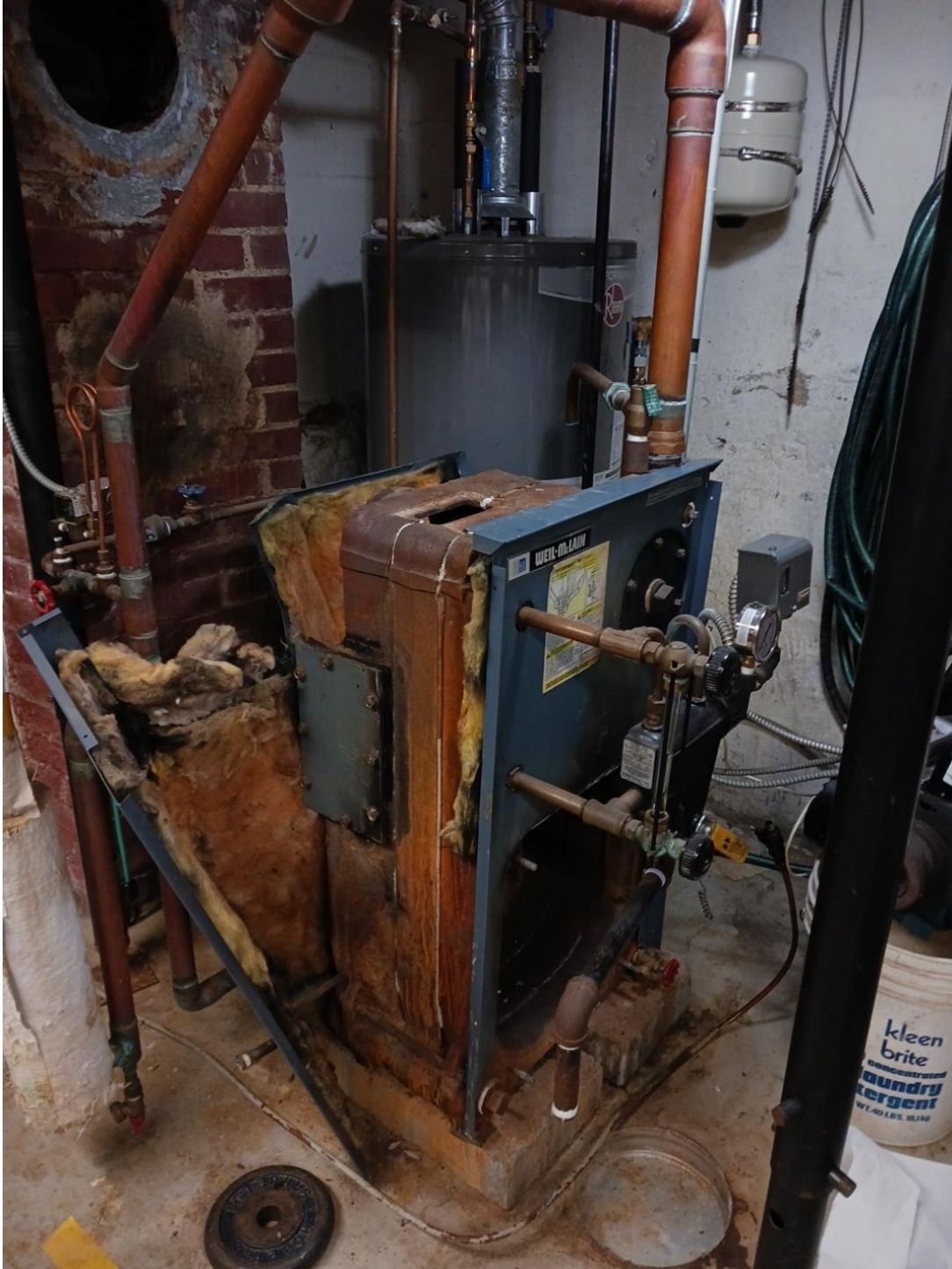
Figure 3 Disassembly of sheet metal shroud. Removal of a few sheet metal screws and alteration of one back section enabled the shroud to be easily removed. Removal of the burner and controls was necessary to remove the front panel, though it was learned that was not necessary for this repair.
