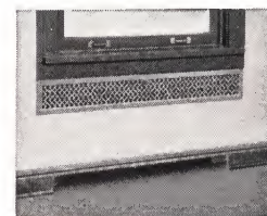
Concealed Radiator, Plaster Front
