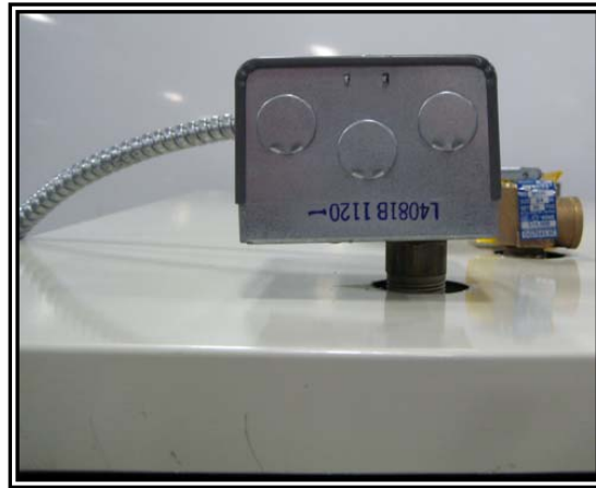
Figure 7: Aquastat-Immersion Control, Mounted
