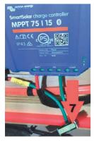
The solar charger is mounted on the rear bulkhead of this compartment and if the bright blue doesn't catch your eye, it also flashes blue periodically. There are three possible circuits marked BATT, PV and LOAD. BATT is protected by Fuse #1. Fuse #7 is in-line and protects the PV (Photovoltaic) circuit with a 30-amp ATO. Fuse #8 is hard to see because its physically mounted on the
