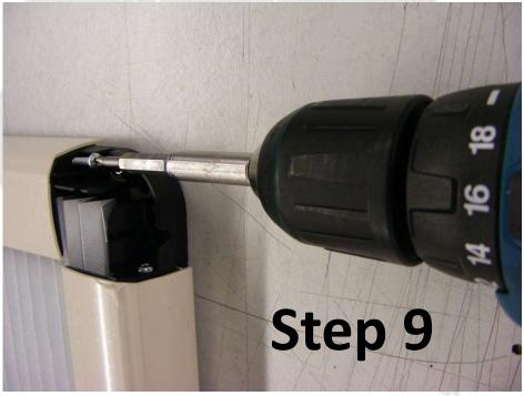
Fasten the corner pieces to the side profiles using the screws provided in the hardware kit. Repeat this for all four corners.
