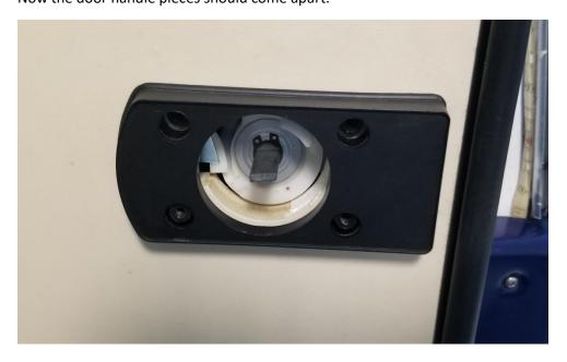
Remove the screw on the silver piece on the right. Note the direction for it to go back together.
