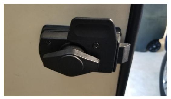
Use a very small screwdriver and pop out the center button on the handle to reveal the screw. Don't do like me, thinking it just snaps off and mutilate it.
