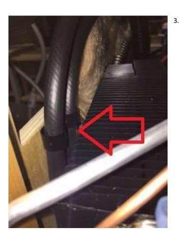
This is an example of the proper installation of the gas hose with clips. The hoses do not touch the 3-way refrigerator fins.
