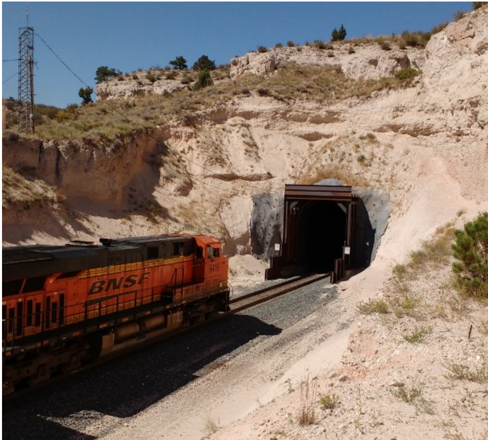
Tunnel # 1 East Portal West Bound Train
